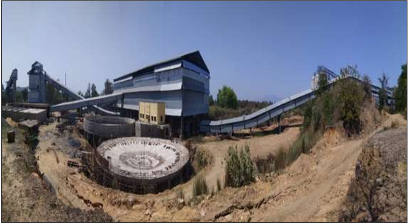
Washery Building with Thickener
