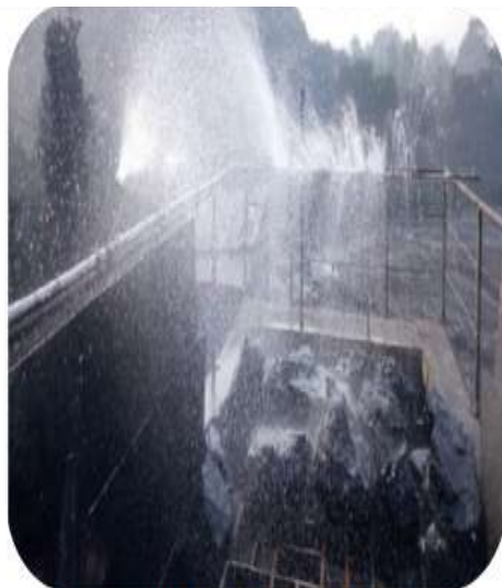
Fixed sprinkler at Coal Crushing point
